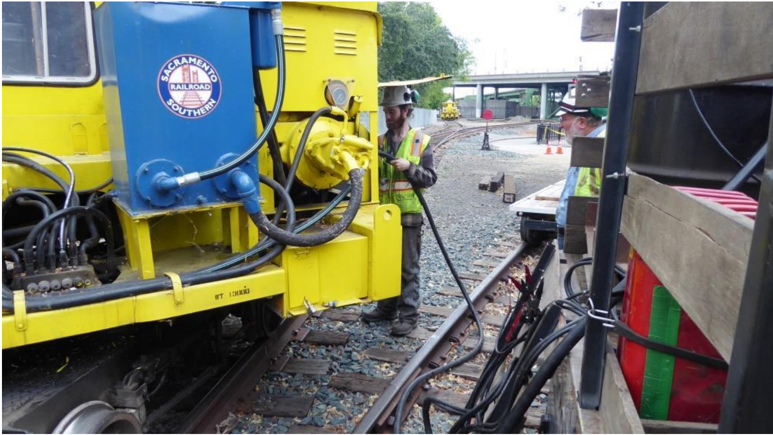
Next up, Matt and Frank fuel the tie-crane
