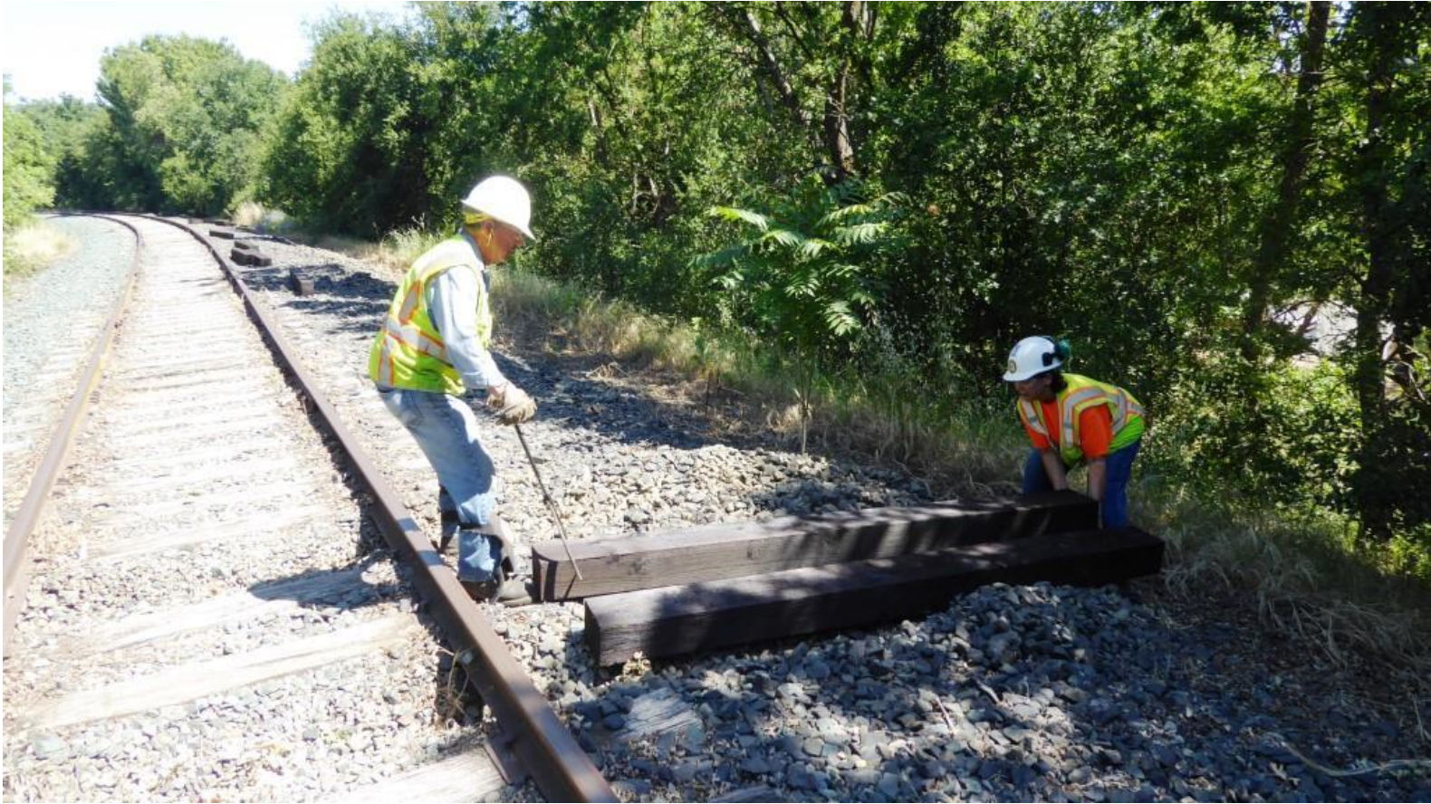
Mike T. and Pam position new ties along empty tie-cribs...
