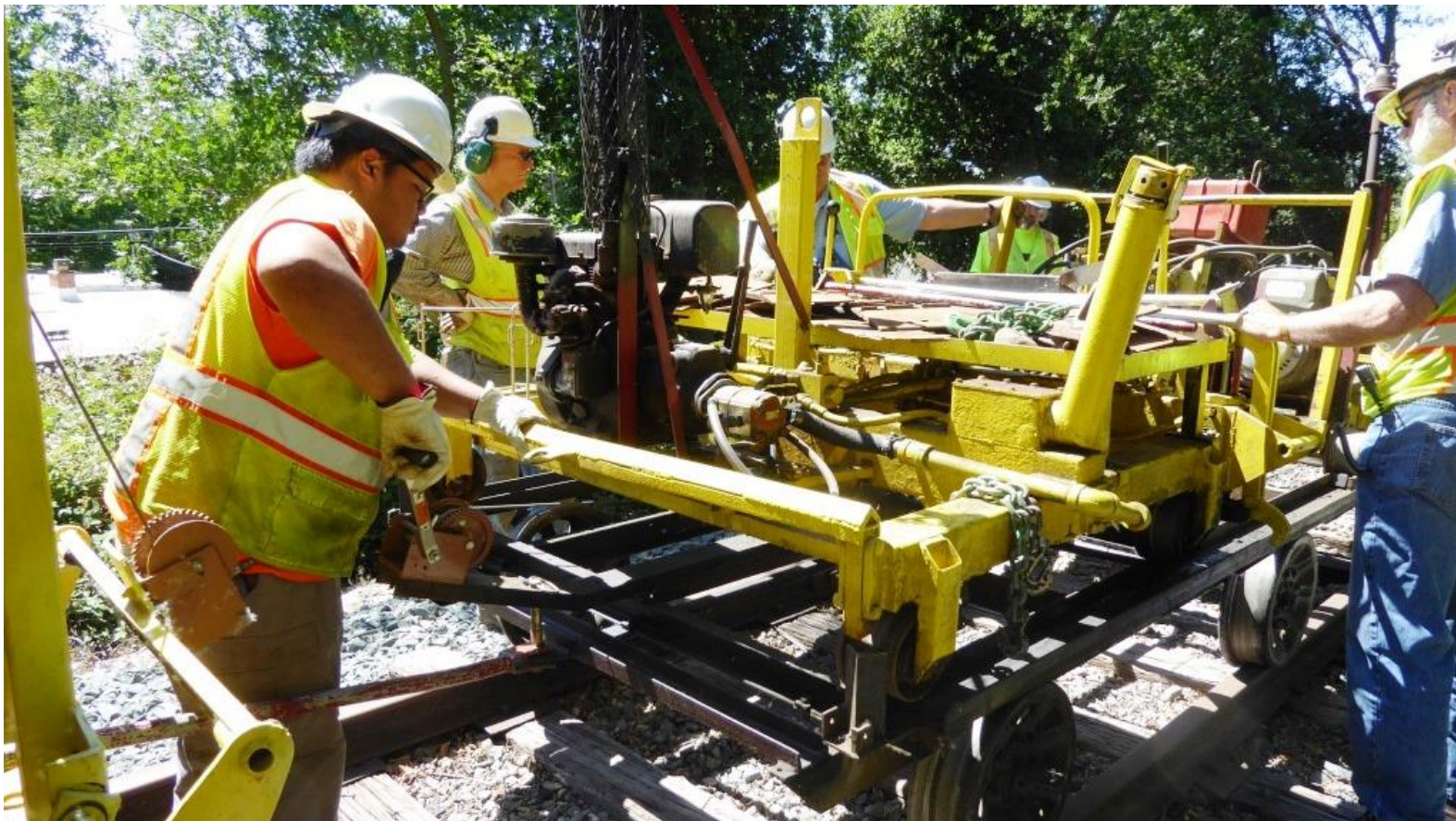
Anthony cranks on the hand-winch and pulls the gauger back into position on its carriage
