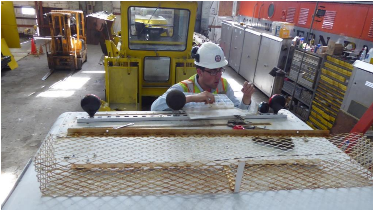
Weston installing a new horn on the Jackson 125 tie-exchanger
