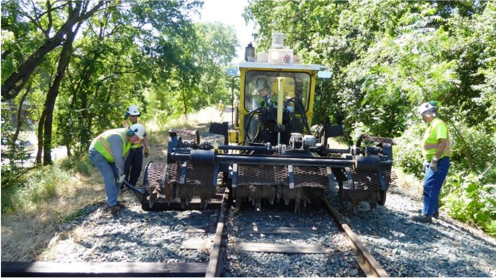
Heather in the scarifier-inserter inserts new ties assisted by Ed M., Steve, and Ed K.
