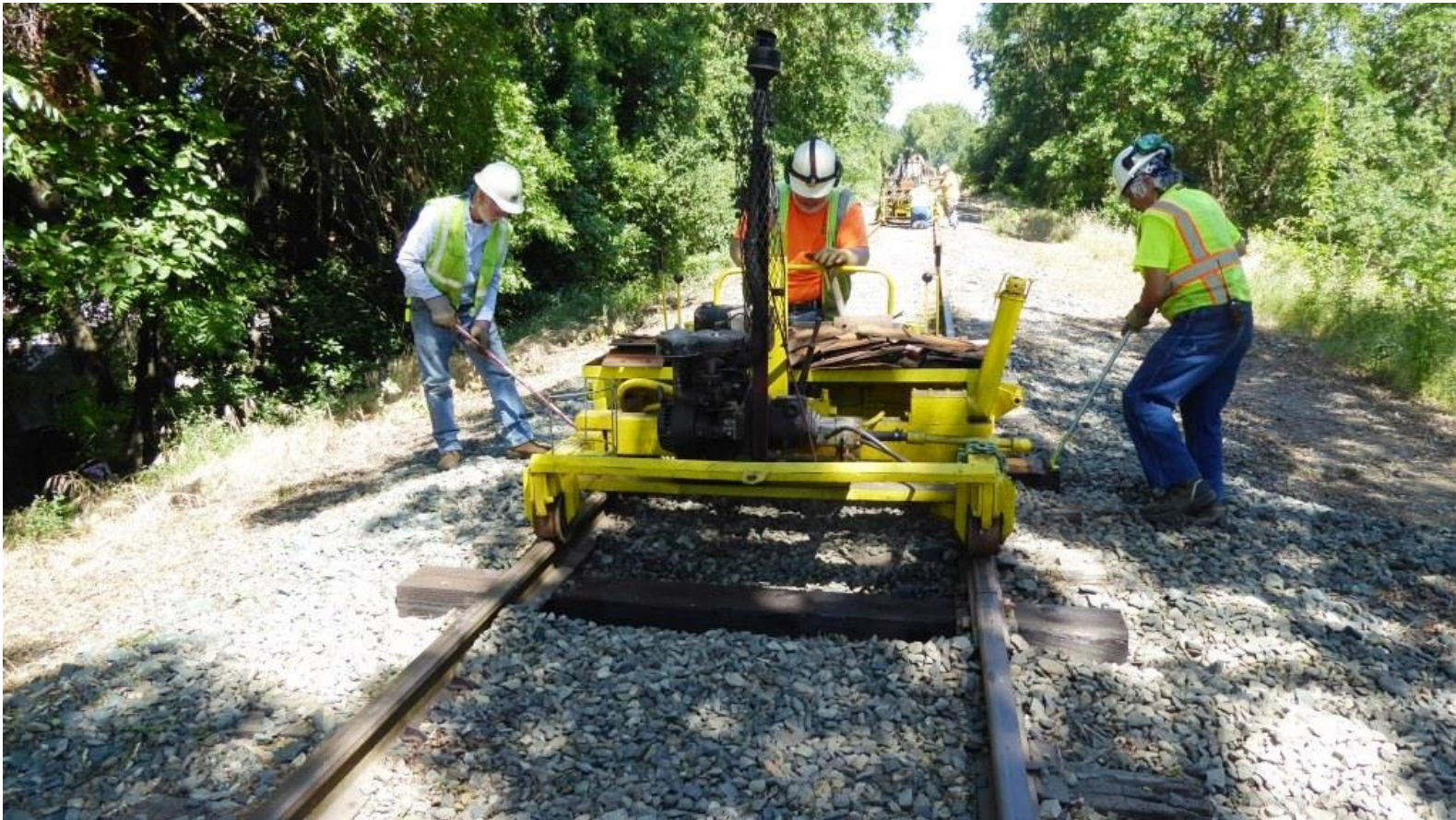
The plate-lifter grabs the rails and lifts them just enough to squeeze tie-plates between them and the ties
