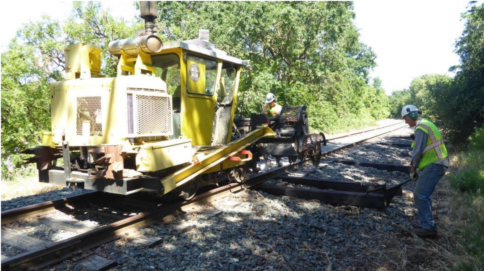
Tie insertion continues with Steve and Ed M. working with Heather in the scarifier-inserter
