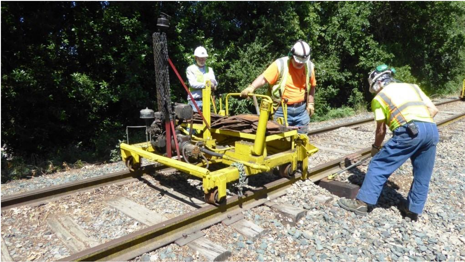
But, the plate-lifter is working as Mike M., Frank, and Ed K. place plates between the base of the rails and the tie
