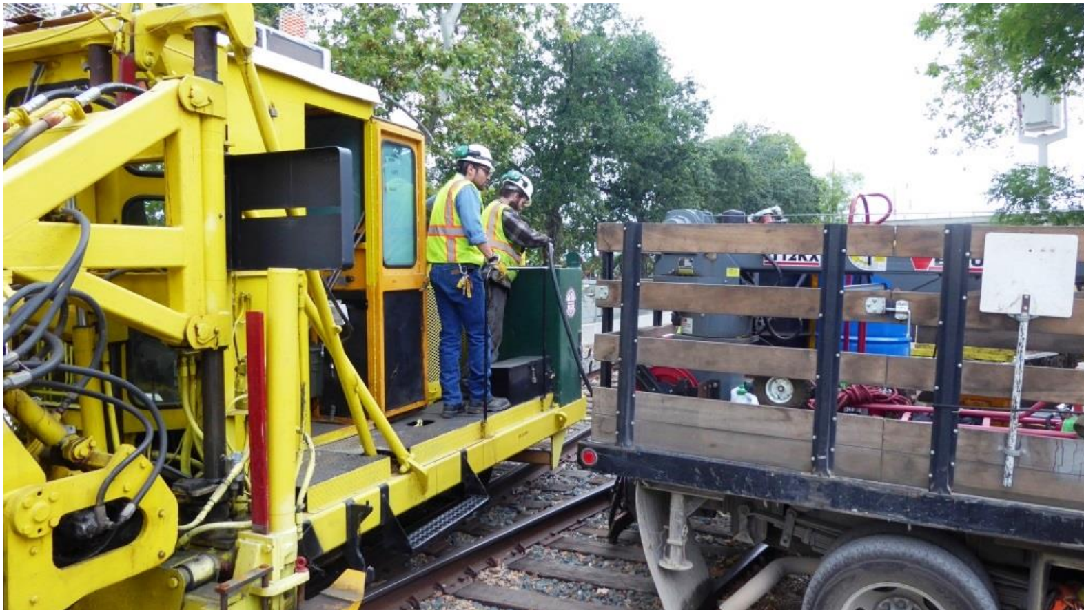
Finally, the tamper gets its tank filled by Kyle and Matt
