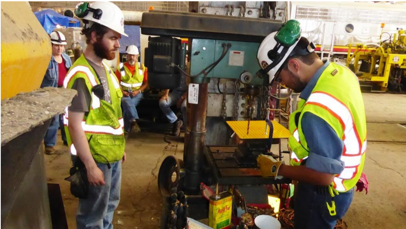
Matt and Kyle drill bolt-holes in the new switch targets
